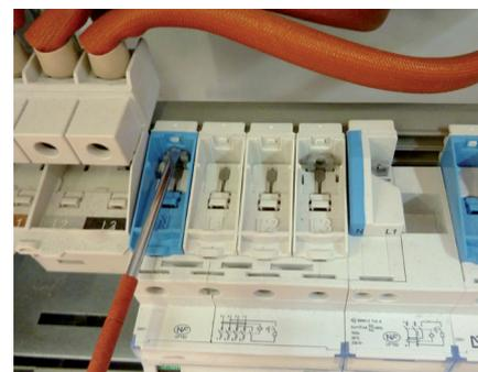
Installation is complete once all the clips are in the locked position.
