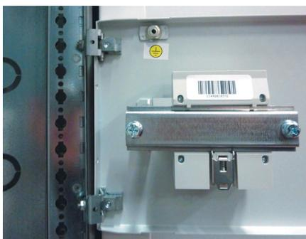
After screwing both hinges onto the faceplate as indicated in the instructions, fix the assembly on the faceplate support upright using the two nuts supplied.
