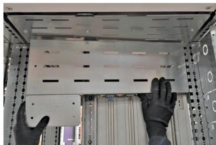
Similarly, for the front of the enclosure, a 200 mm plate is provided. Depending on the height of the busbar, one or two 100 mm additional elements can be added on the right-hand side of the column chassis.
