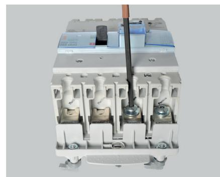
Make the upstream electrical connections with the screws supplied with the circuit breaker (no. 4 Allen key, tightening torque 7 N·m).
