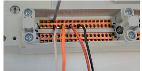
Once the MCCB is in position, connect the wires to the module for auxiliary circuits, on the movable part of the base. The connection module has screwless terminals and the use of Starfix ferrules is recommended for wiring.
