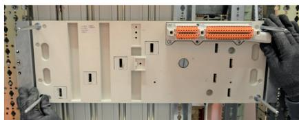
This part hooks onto the uprights just like an ordinary plate with its metal lugs.
