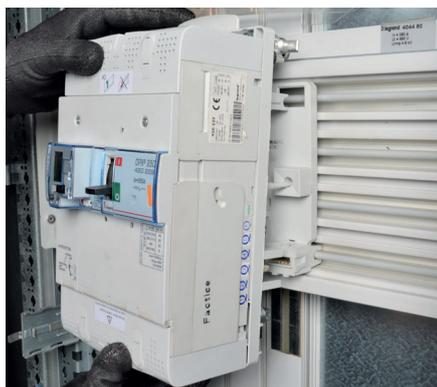
Guide pins make it easier to insert the circuit breaker equipped with the movable part.
