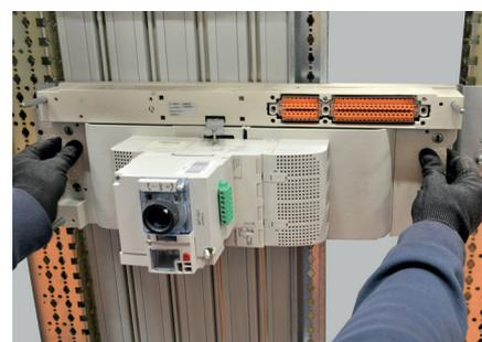
The movable part is inserted in the fixed part using the four metal guide pins.
