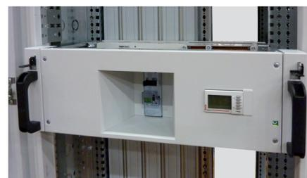
Once assembly is complete, the measuring device can be wired up to the tray connector in the same way as for the circuit breaker auxiliaries using the free terminals on connector B.
