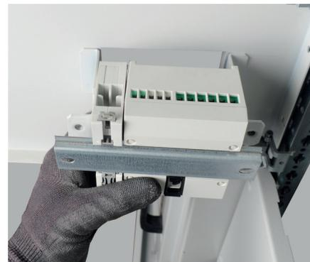
Install the modular device on the DIN rail.
