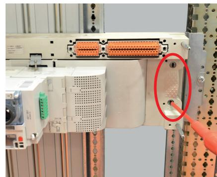
The movable part is locked onto the fixed part using the 1/4 turn screws (two on each side).
