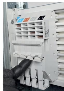
Complete installation of the support base by closing the locking levers. Once locked onto the distribution block, the support base allows the circuit breaker to be installed in the same way as on a standard DIN rail.
