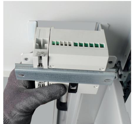
Open the pre-cut window in the faceplate, then install the modular device on the DIN rail.
