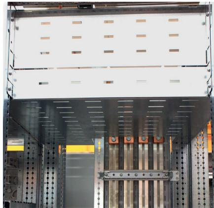
The divider for the horizontal busbar must be completed with a backplate. This divider is supplied for 400 mm high partitioning but can be adapted to 200 or 300 mm.
