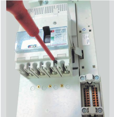
Place the device in the drawer and secure it with the two screws supplied with the circuit breaker (tightening torque 1 N·m).
