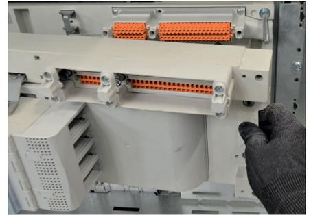
Insert the movable part equipped with the circuit breaker in the fixed part using the four metal guide pins.
