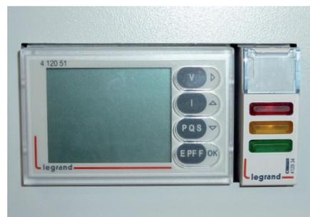
The faceplate allows a modular device, such as a measuring device, to be installed (see page 45). It is also possible to install led lights.
