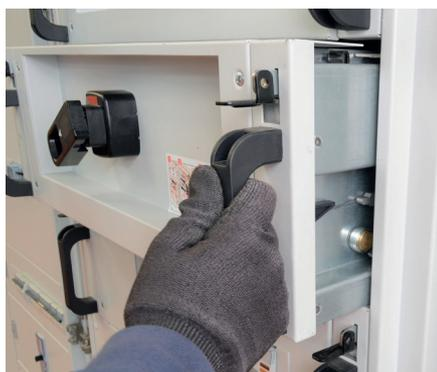
Hold the tray against the fixed base and push as far as the locking hole. The tray is then in the removed position, with the upstream and downstream main contacts disconnected and auxiliary contacts disconnected.
