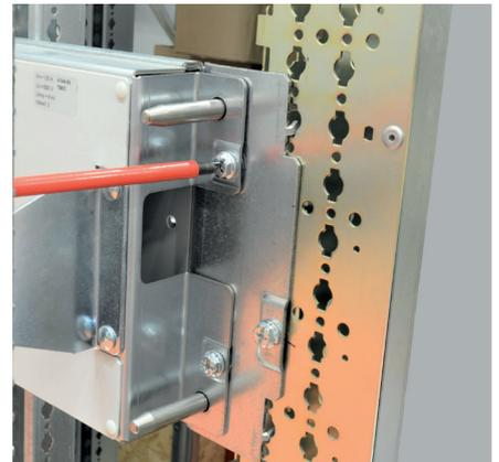
Fix the movable part to the fixed part with the screws supplied.
