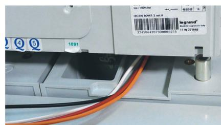
When installing the circuit breaker, space is left on the base to allow the wires to exit.
