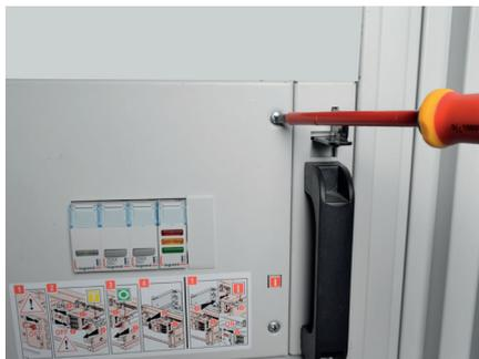
Position the faceplate and tighten the four screws.
