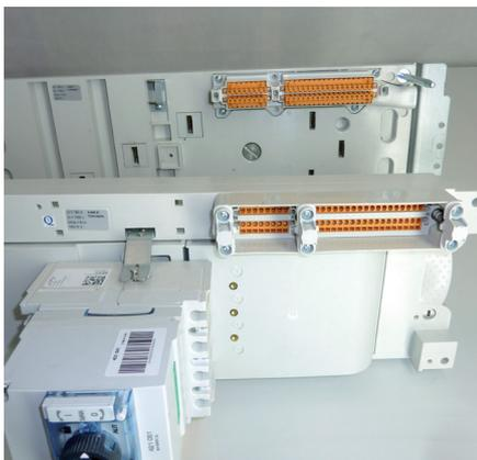
Place the male part of the connection module on the fixed part of the VX<sup>3</sup> IS base and the female part on the movable part using the screws supplied.
