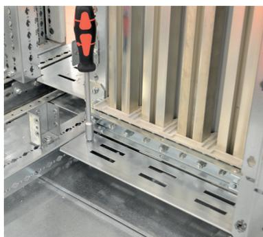
The top and bottom cover plates are screwed onto brackets before the side partitions are inserted.
