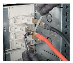
IS 233 bases are connected downstream using bar ends with two drill holes for M8 screws, enabling connection via bars or lugs.
