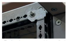
The faceplate support uprights are fixed in the first tapped hole 50 mm from the front (below the earth symbol).
