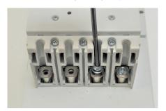
Tighten the upstream and downstream electrical connections using the eight (or six) screws supplied with the circuit breaker. Apply a tightening torque of  $7 \, \text{N·m}$ .
