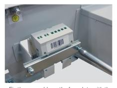
Fix the assembly on the faceplate with the screws supplied.
