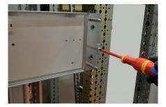
Then secure the fixed part using the screws supplied with the row distribution block.
