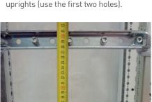
Intermediate supports are then fixed every 300 mm (tightening torque: 15 N·m).
