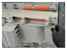
Insert the movable part equipped with the circuit breaker in the fixed part using the four metal guide pins.
