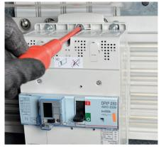
Complete installation of the DPX3 by locking the 1/4 turn screws above and below the circuit breaker.
