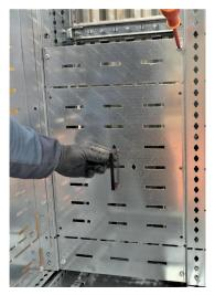
The cover plates are manipulated with a removable handle supplied in the kit. They are screwed onto the side partitions.
