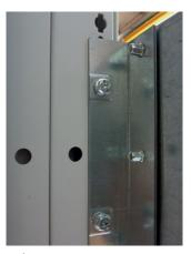
Fix the base to the functional uprights (10 N·m) then to the uprights on the front of the structure using brackets (4 N·m).
