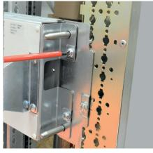
Fix the movable part to the fixed part with the screws supplied.
