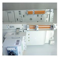
Place the male part of the connection module on the fixed part of the VX3 IS base and the female part on the movable part using the screws supplied.
