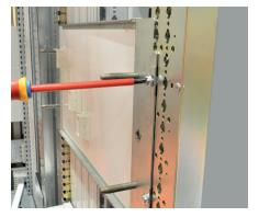
Place the fixed part in position and fix it on the IS chassis functional uprights.
