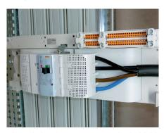
Install the downstream terminal shield, and insert both locking caps (in this photo, the circuit breaker has a rotary handle).
