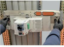
The movable part is inserted in the fixed part using the four metal guide pins.
