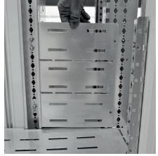
By default, spare compartments must be fitted with dividers (Cat.No 4 046 89) which can achieve form 3b, the minimum level required for IS 233.
