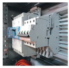
New circuit breakers can be added with the voltage present as long as the panel is off-load (circuit breaker in open position), like all products in the IS range.
