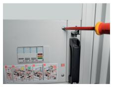
Position the faceplate and tighten the four screws.
