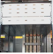
The divider for the horizontal busbar must be completed with a backplate. This divider is supplied for 400 mm high partitioning but can be adapted to 200 or 300 mm.
