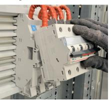
Engage the MCB in the same way as onto a standard DIN rail.
