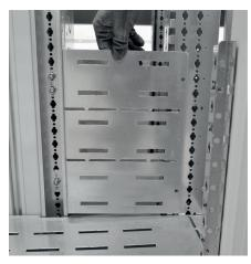
To obtain form level 3b, the part of the IS chassis not equipped with the VX3 IS base must be closed at the front with 300 mm high spare compartments Cat.No 4 046 89. If necessary, they can be cut at 100 mm intervals.
