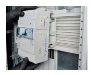
HX3 IS 250/400 A ROW DISTRIBUTION BLOCKS This allows unstream connection/disconnection with the voltage present (circuit breaker open: circuit off-load) and the mix of DX3 and DPX3 circuit breakers
