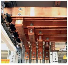
Mounting connection kit Cat.No 4 046 91. Tightening torques:
