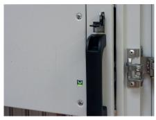
The tray position is indicated by a coloured LED and can be locked out with a padlock.
