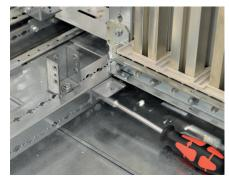
Also fix the four brackets for the top and bottom cover plates 325 mm from the front.
