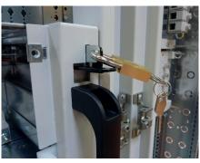
Locking the drawer in each of the three positions is possible with a ordinary padlock maximum diameter 5 mm (for example ref. 4 063 13) inserted at of the locking lever. A location is available on each of the two levers.
