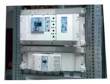
DPX and DPX3 circuit breakers are mounted horizontally on the bases.
