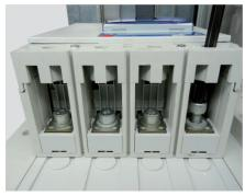
Tighten the upstream and downstream electrical connections using the eight screws supplied with the circuit breaker. Apply a tightening torque of  $24\ N\cdot m$ .
