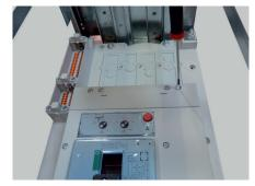
Fix them using the screws supplied (two per terminal shield).
