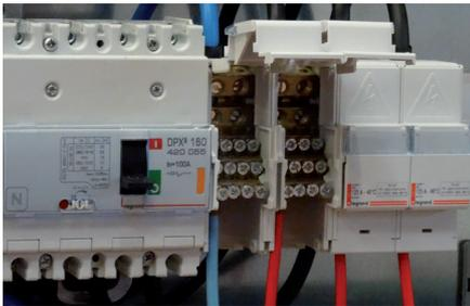
Modular single-pole distribution blocks: total isolation of poles in order to distribute up to 250 A (160 A max. in a XL<sup>3</sup> 160 cabinet)
