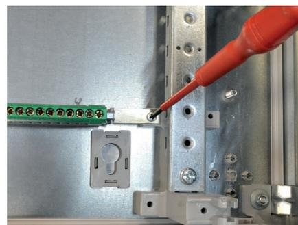
Fix the bar on the plastic supports integrated at the back of the cabinet
