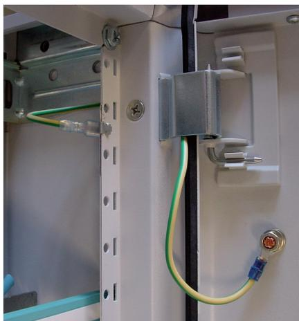
Conductor Cat. No. 0 373 85 clips directly onto the faceplate support inside the enclosure
