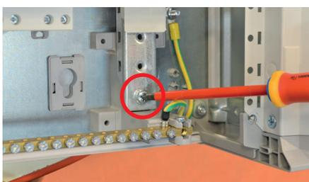
With the faceplates removed, the chassis can be removed from the cabinet after unscrewing the 4 retaining screws (one at each end of the chassis)
