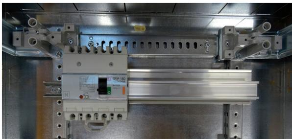
Photo with rail in a low position equipped with a DPX<sup>3</sup> 160 and a height spacer Cat. No. 4 052 26
